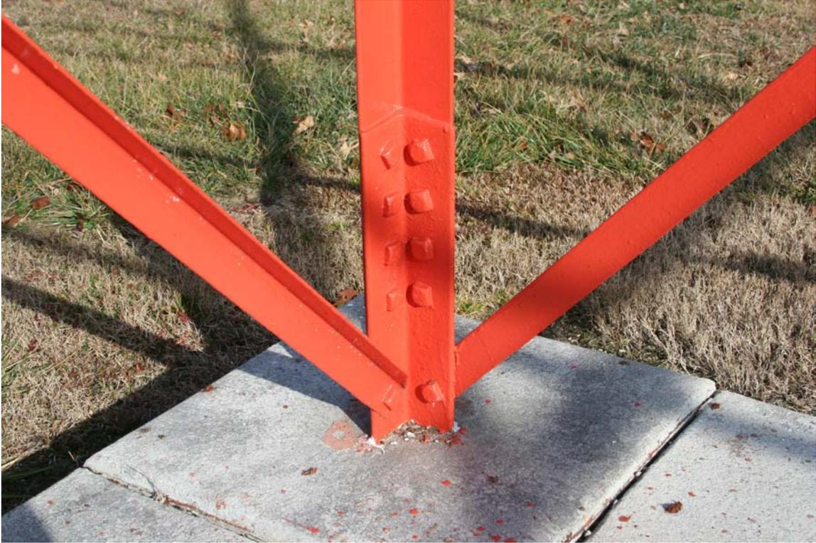
Close up of the base of the Crossville, TN airport beacon showing the stub set in concrete with the tower attached to by 4 bolts and a single bolt for brace attachment.
