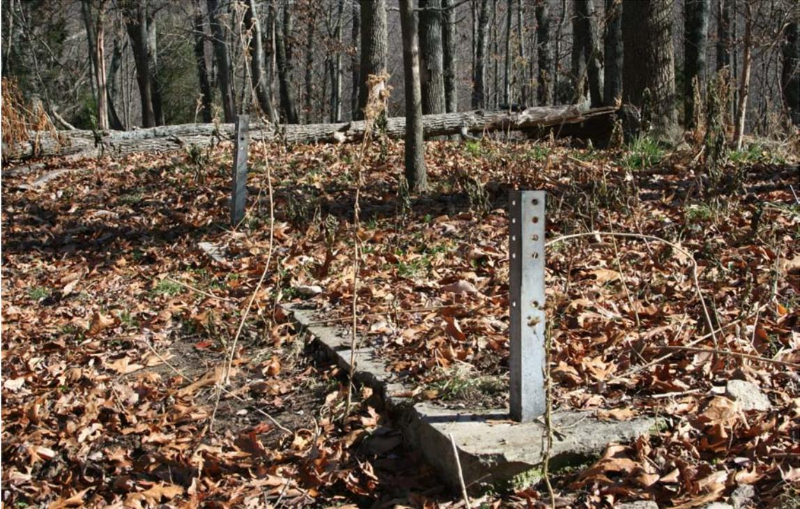
Another view of the base, showing how the legs were set in a concrete footer. The legs have 4 bolt holes for tower attachment and a single hole lower down for a brace attachment.
